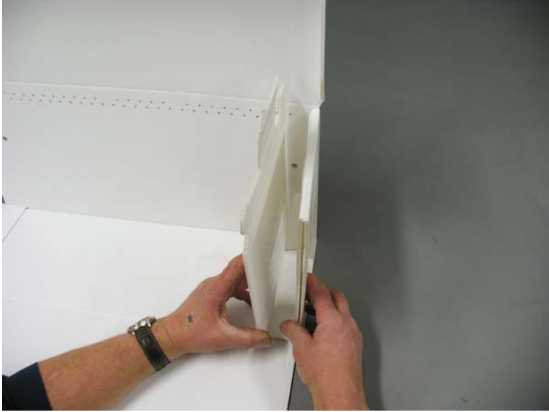
Form bottom corner of ventilation section
