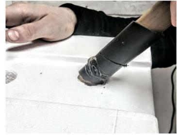
7. Assemble 17/64" drill bit and drill. Using plywood shim provided with predrilled hardware hole as a guide, drill hardware hole in affixed entrance shims.
